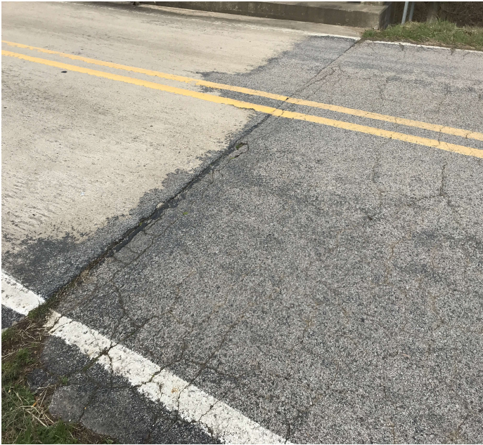
PHOTO 1 Description East approach minor achm settlement.
