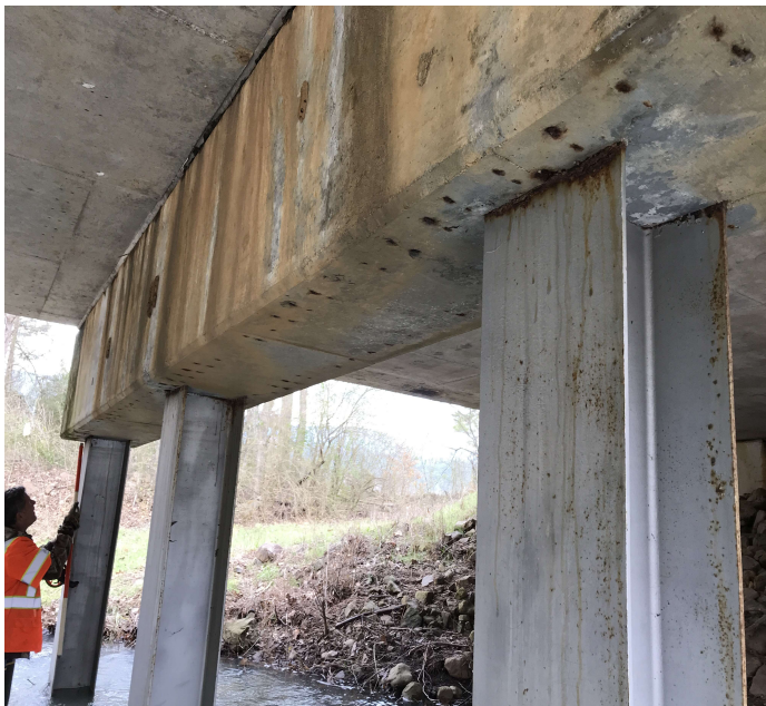
PHOTO 1 Description Bent # 3 active corrosion with minor section loss at the cap juncture.
