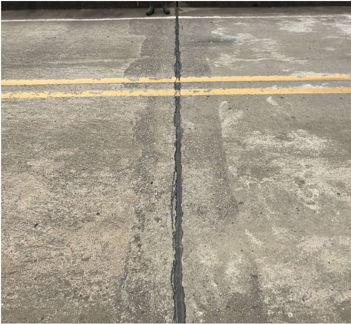
PHOTO 1 Description Bent # 2 joint seal adhesion failure.
