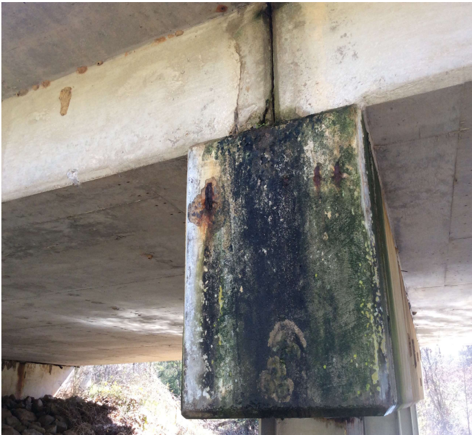
PHOTO 1 Description North end of Bents 2 & 3 caps have minor golf ball size spalls with exposed reinforcing steel.
